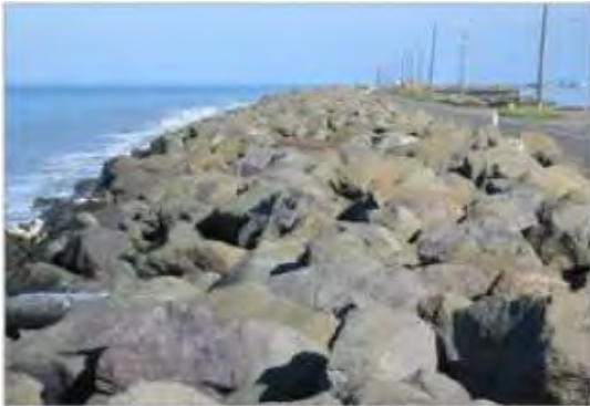
Riprap on Ediz Hook in Port Angeles
