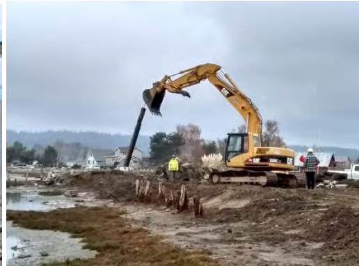
Maylor Point tire wall (one of several types of hard armoring) before and after removal. Credit: Lisa Kaufman
