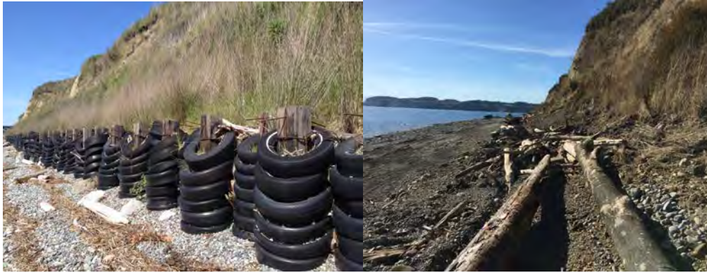
Maylor Point tire wall (one of several types of hard armoring) before and after removal. Credit: Lisa Kaufman
