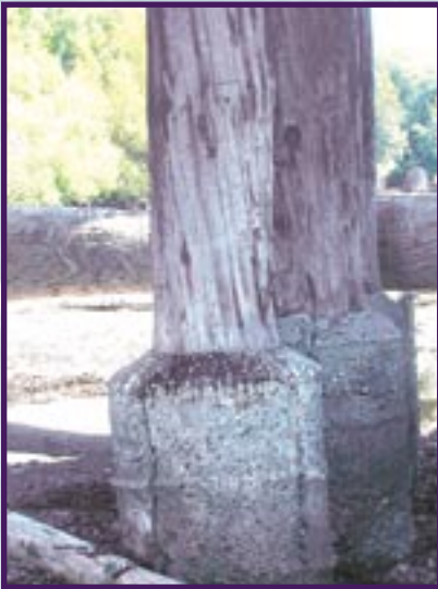
Creosote leaks out of old pilings in the intertidal zone, leaching toxins directly into the water and surrounding substrate.
