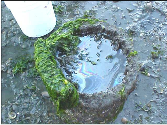
Figure 1. Creosote compounds leaching from an old piling in South Fidalgo Bay. Photo by Paul Dinnel.
