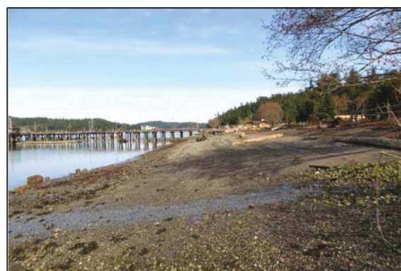
Figure 4. Photo of restored shoreline taken at on March 4, 2013. Bulkhead and fill removed and shoreline topography restored to enhance nearshore habitat for fish and other species.
