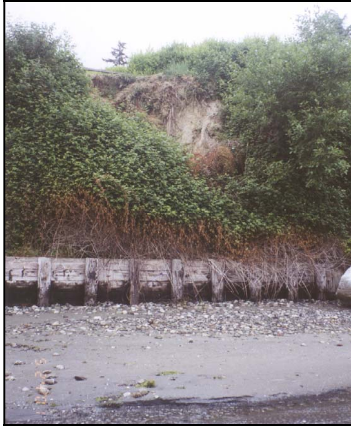
Figure 11: Structures are often intended to prevent erosion or to provide people with access to the shoreline. Both types of structures can negatively impact nearshore habitat, especially as the structures begin to fail.
