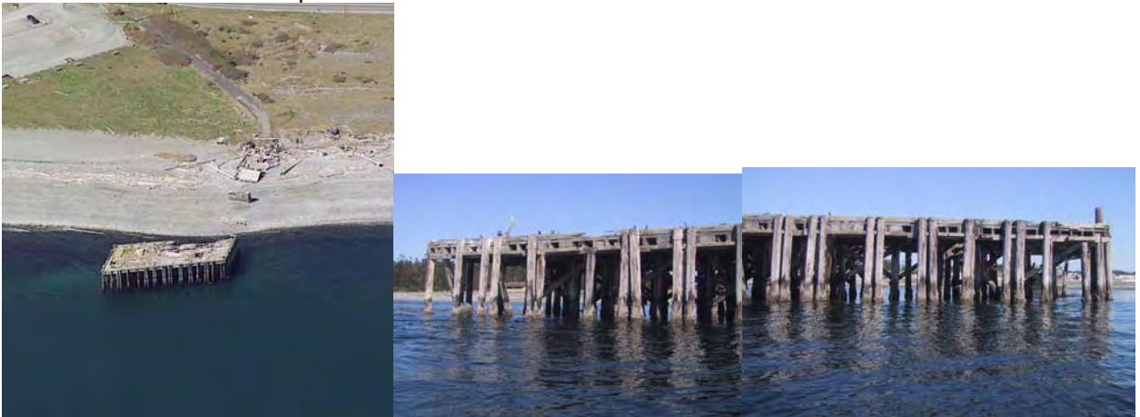
71 Remove 115 creosote piles from old structure in subtidal
