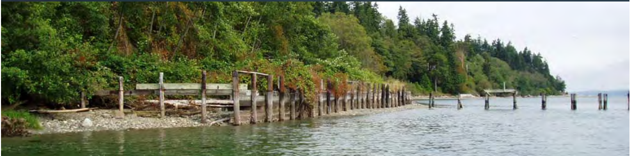
44 Remove failed pier and creosote piles
