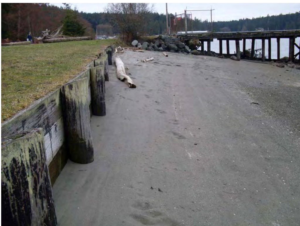
Figure 5. Accumulation of sediment on the northeast side of the Marine Maintenance and Facilities Dock. Fill associated with the dock approach protrudes into the intertidal area. March 27, 2009.
