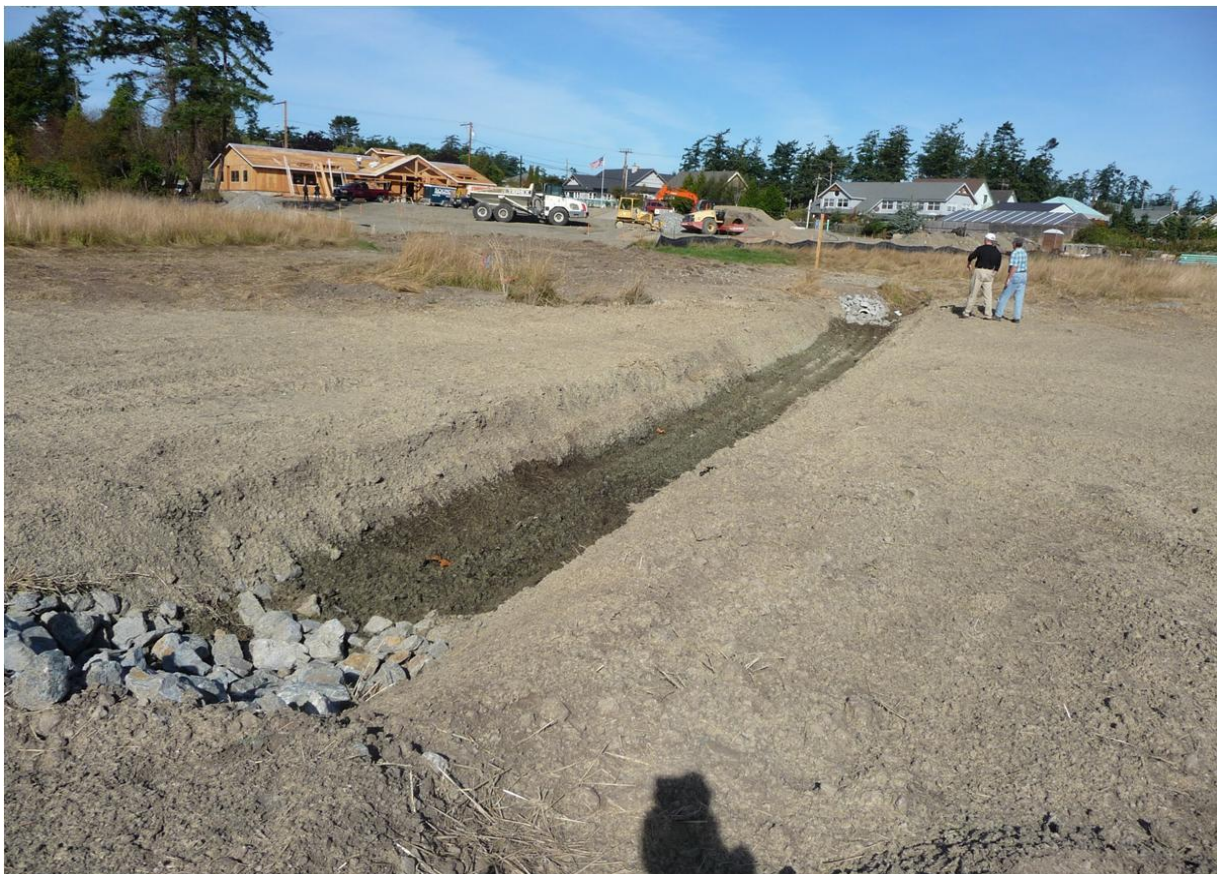
Figure 9: South Drainage Ditch EBuffer Tile Drain or Overflow (Photo 9.19.09)
