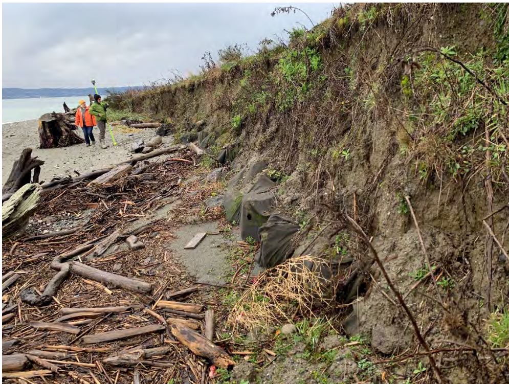
Figure A-9. Looking south at erosion and exposed geotextiles.
