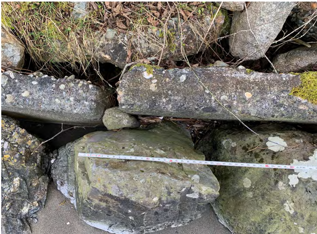
Figure A-4. Example of armoring along the shoreline.
