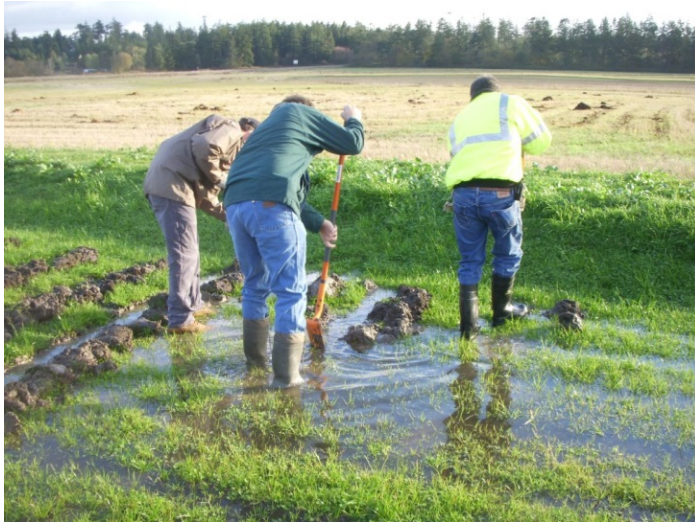
Figure 1-2. Digging trenches for tree planting in the swale.
