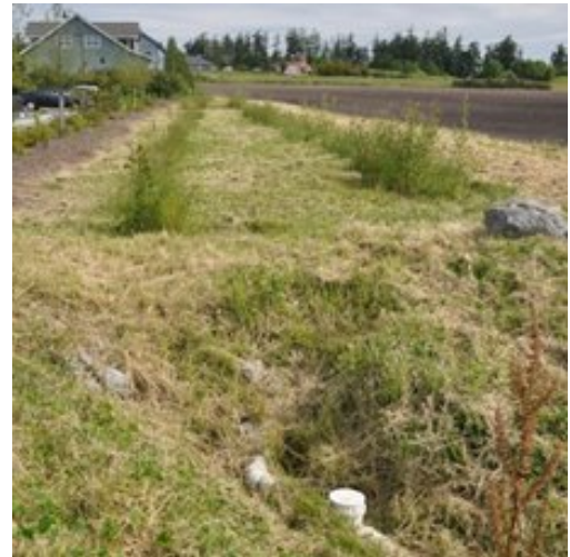
Figure 1-3. Swale including underlying drain pipe outlet.
