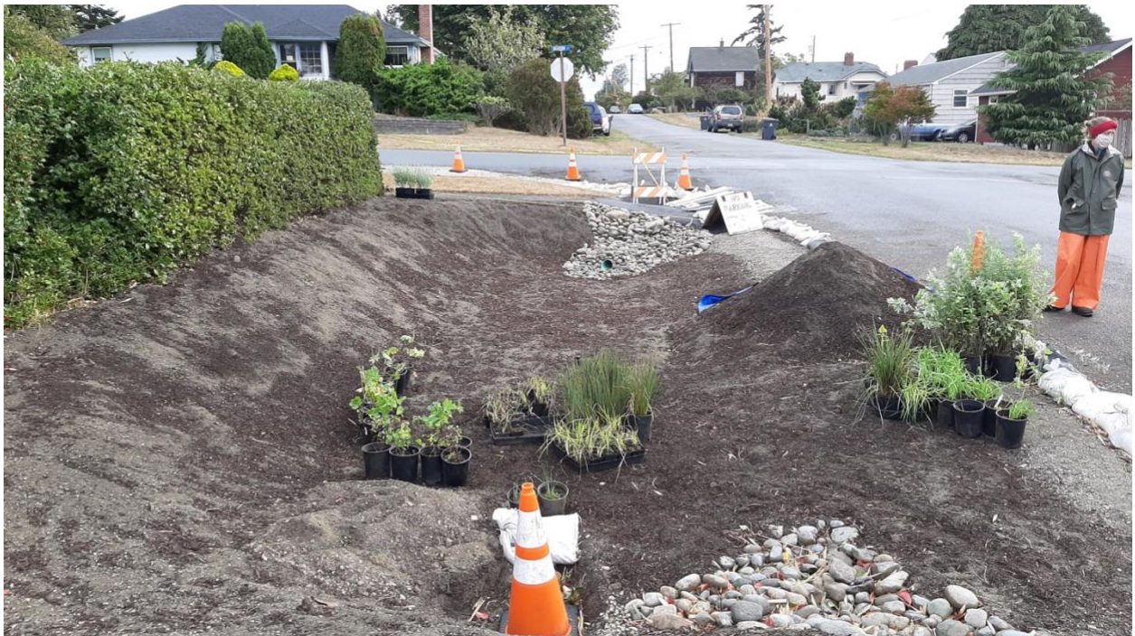
Second rain garden installation: Benton & Clay Streets in Uptown Port Townsend
