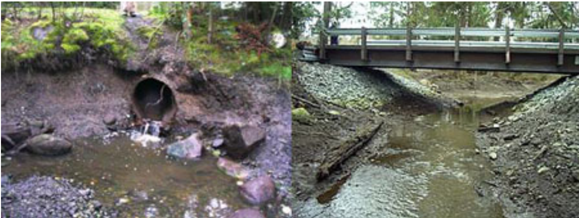
Figure 1. In September 2006, a culvert was replaced and a bridge was installed. The before and after restoration pictures above were taken at low tide.
