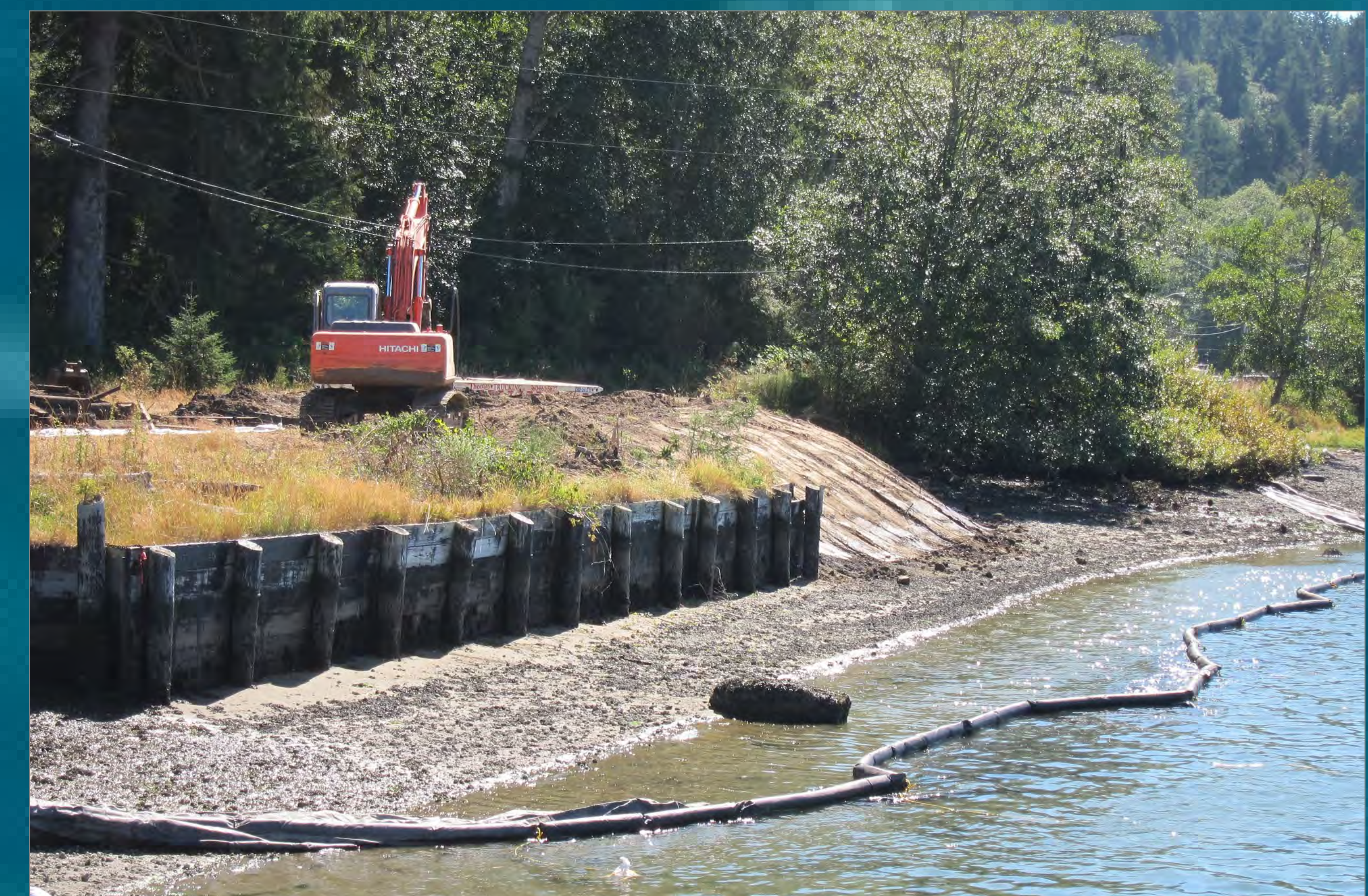
The construction phase of the beach restoration at Cornet Bay, removing creosoted bulkhead from 800 feet of shoreline.
