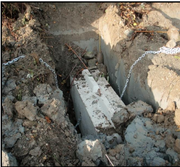
Ecology block with chain to hold logs in place. Photo # 7
