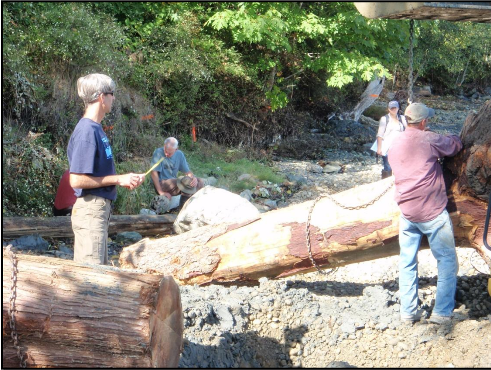
Moving root wad into place. Photo #6
