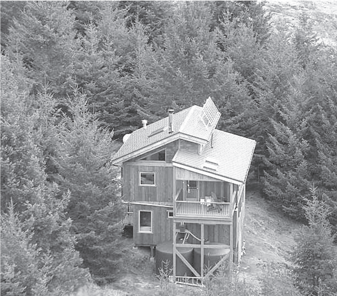
Photovoltaic panels provide power and roof catchment provides water for off-grid home. Photo by Rainshadow Solar
