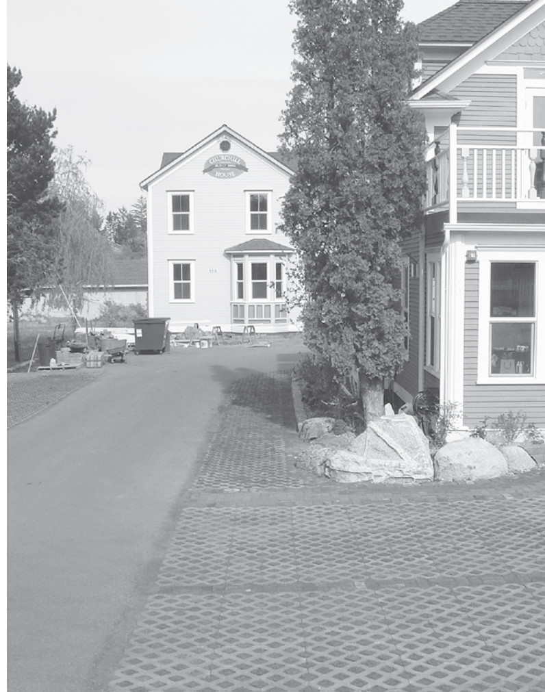
Pervious pavers installed by Archipelago Properties filter stormwater and return water to the aquifer. Photo by Liz Illg
