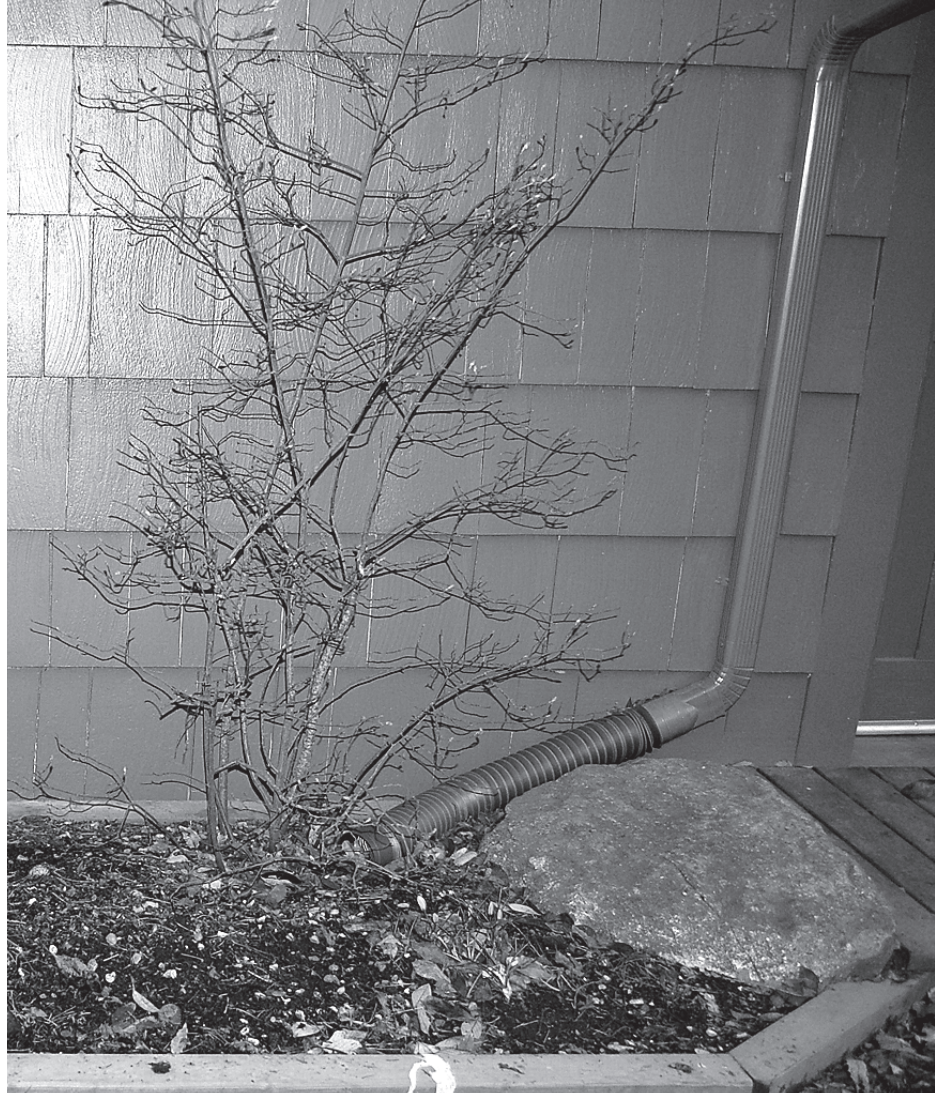
Capturing and diverting rainwater in Eastsound. Photo by D. N. Kinsey, ASLA
