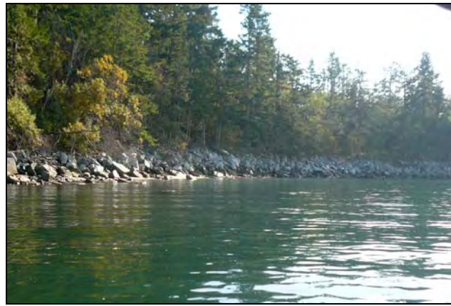
Figure 15. Armored (historic) feeder bluff along Shannon Point shore.
