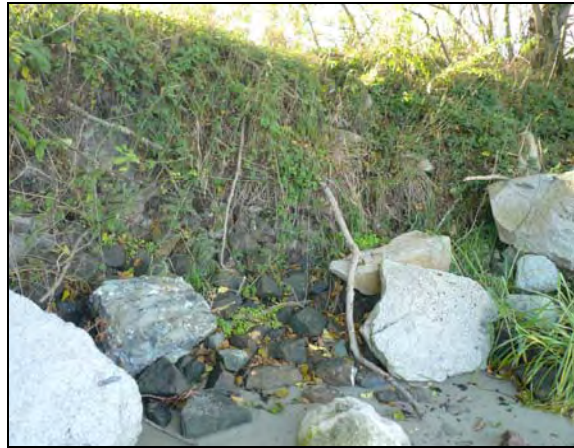
Figure 19. Armoring at base of dike/fill that impounds Cannery Lake wetland.
