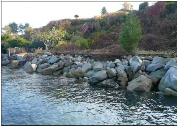
c) Modified by historic rail revetment
