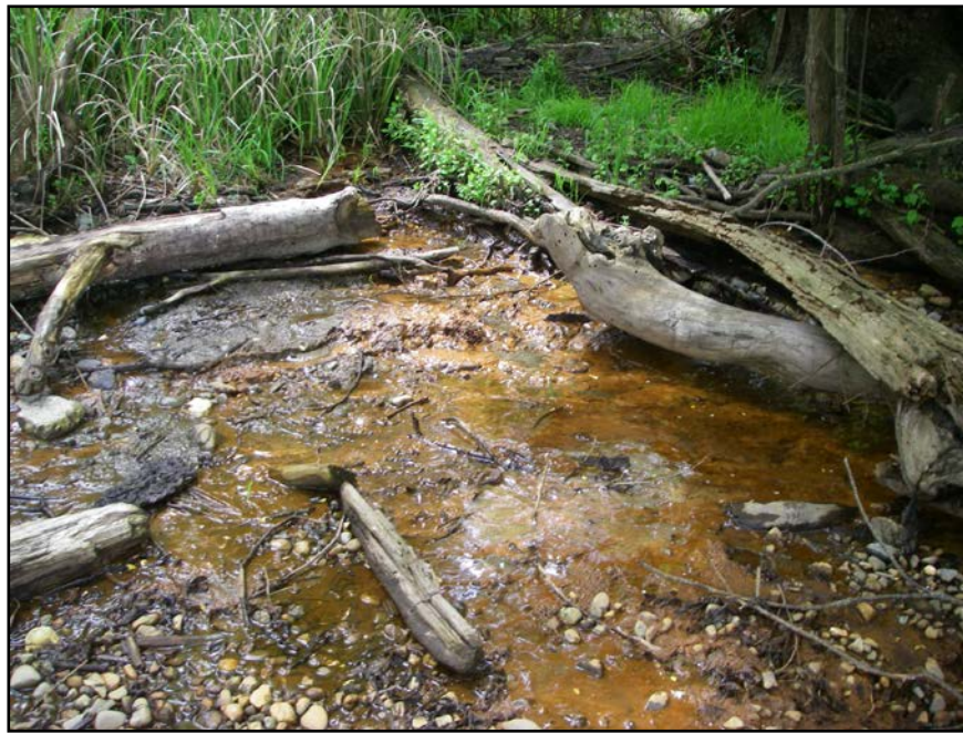
Figure 18. Guemes Channel side of the railroad berm (top) showing the approximate water level (about 1 meter above the upper shoreline -- white dashed line) in Cannery Pond behind the berm. The bottom photo shows an area of seepage through the berm on the west end of the fill area. Seepage was estimated at about 1 to 2 liters/minute.
