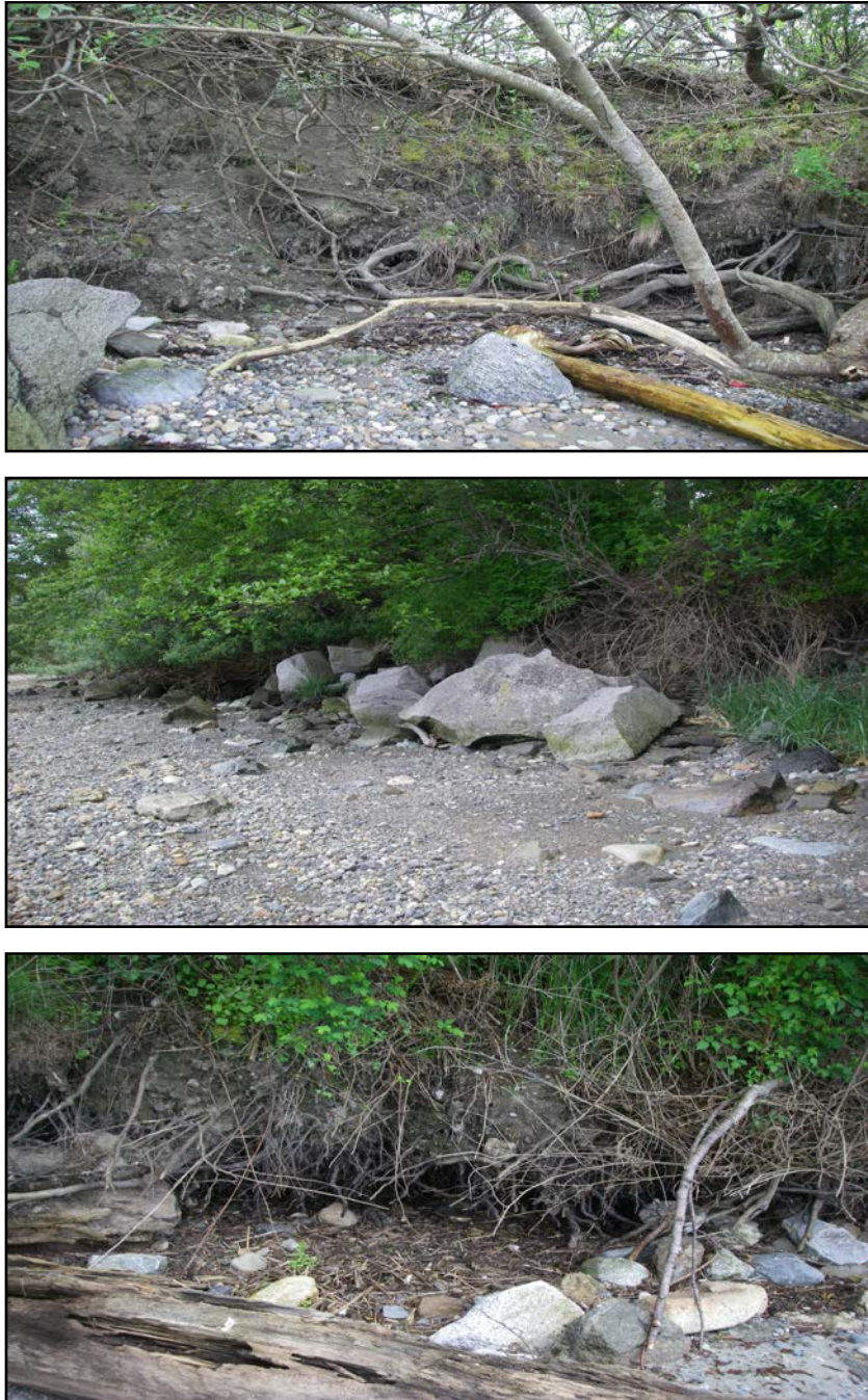
Figure 16. Series of photographs of the Guemes Channel side of the railroad berm showing the unconsolidated nature of the filled area that has been eroded as much as 3-4 meters in places (top), the presence of some riprap (middle) and undercutting of the berm caused by wave action (bottom).
