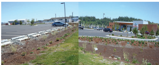
Landscaped bioswales, located at the Anthony's Restaurant parking lot at Cap Sante Marina, absorb the runoff from the parking lot and remove the pollutants left behind by vehicles
