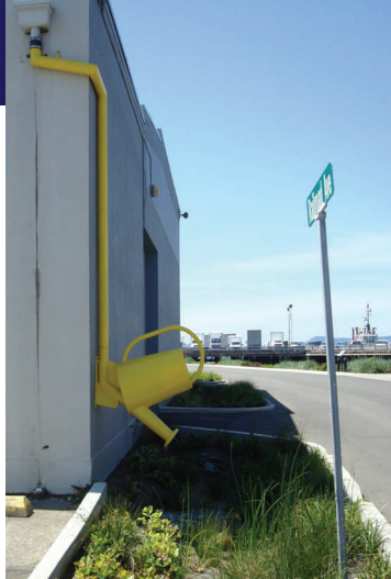
Rain gardens at the Port of Anacortes Rope Building are designed to capture, absorb, and treat roof runoff
