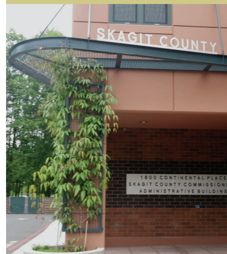
Skagit County Administration Building
