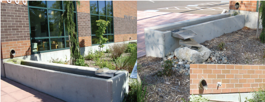
Concrete structures at the Skagit County Administration Building, capture and disperse roof rainwater to the rain garden
