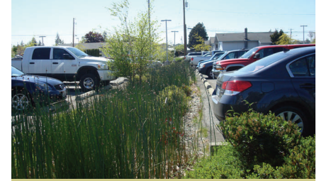
Landscaped bioswales located in the parking lot of the Skagit Valley Hospital absorb the runoff from the parking lot and remove the pollutants left behind by vehicles
