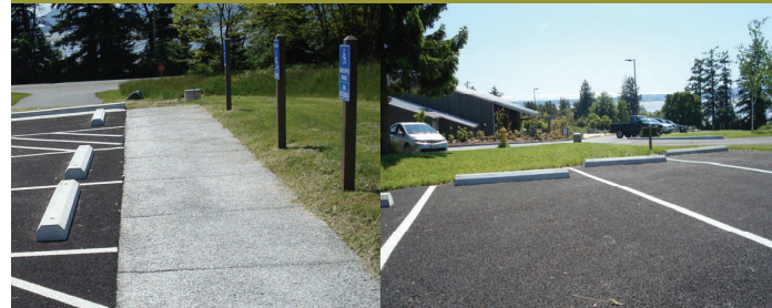
Pervious asphalt parking lot and pervious concrete sidewalk at the Padilla Bay Estuarine Research Reserve allow water to infiltrate and remove pollutants
