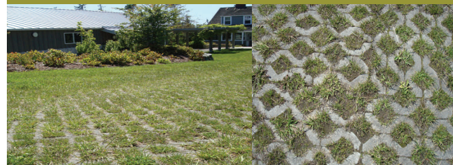
Pervious concrete grid filled with grass at the Padilla Bay Estuarine Research Reserve infiltrates stormwater and provides a durable parking area for vehicles
