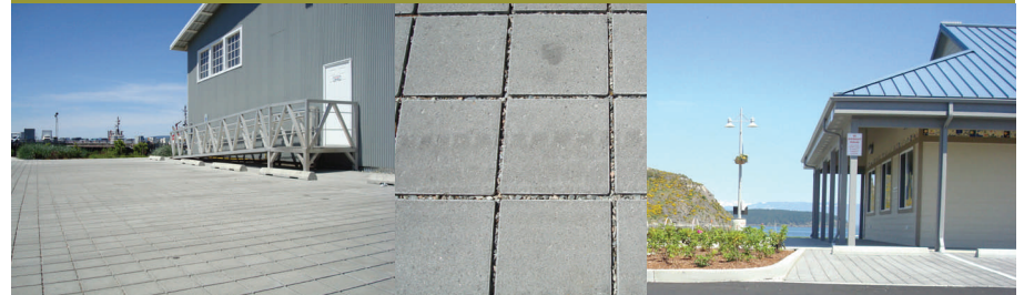
Pervious pavers at the Port's Seafarers Memorial Park allows stormwater to infiltrate through void spaces and gaps between the pavers and into the subgrade layers
