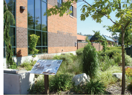
The rain garden at the Skagit County Administrative Building captures, absorbs, and treats roof runoff
