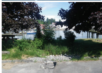
Two rain gardens at the Swinomish Planning Department capture and treat parking lot runoff
