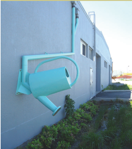
Decorative roof rainwater collection system at the Port's Rope Building captures and disperses roof rainwater to the rain garden
