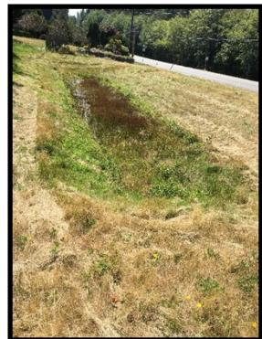
**SWALES:** swales look a lot like a grassy ditches, but they have a purpose! The gentle slope and flat, grassy bottom allows the water to slow down and the dirt to settle out. Some of the water can soak into the ground and what doesn't can continue on its way a little cleaner. Can you find something similar and post it on Instagram **#FidalgoBayDay2020**? **\*Bonus Point:** Find the swales in these pictures located in Anacortes.
