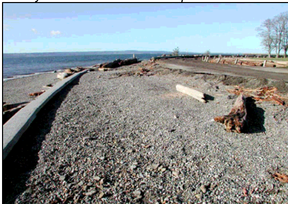
Figure 6. Exposed bulkhead and southwest loop road. Note landward extent of large woody debris following 2/4/06 storm. Photo courtesy of Snohomish County Parks and Recreation Dept.
