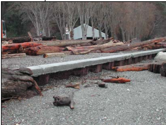
Figure 5. Exposed sheet pile bulkhead along southern shore following 2/4/06 storm. Photo courtesy of Snohomish County Parks and Recreation Dept.
