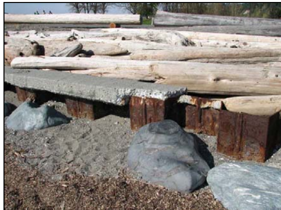
Figure 4. Exposed sheet pile and concrete cap bulkhead following 2/4/06 storm, which was previously buried. Photo courtesy of Snohomish County Parks and Recreation Dept.
