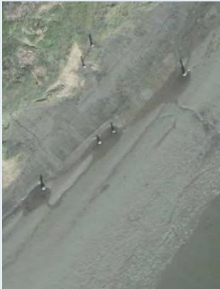
Scour hole depressions visible around pilings
