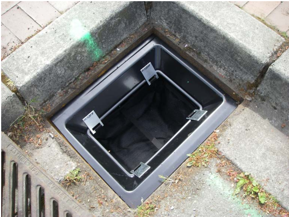
Figure 6. Smart Sponge ® filter unit installed at the Depot in Anacortes, 29 April 2009.
