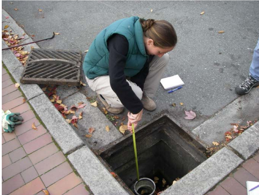
Figure 3. Measuring a storm drain for a Smart Sponge ® storm drain filter.
