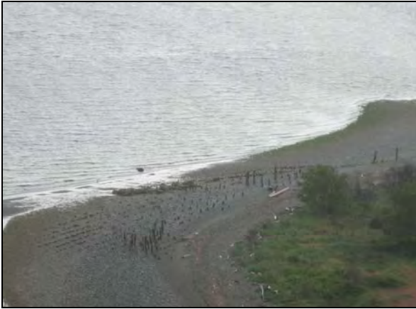
Figure 21. Lily Point piling field (CGS field photo).
