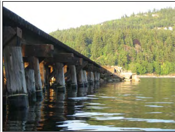
Figure 20. Chuckanut Bay causeway opening, creosote pilings (CGS field photo).
