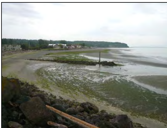
Figure 12. Looking east at armored culvert extending across shore (CGS field photo).
